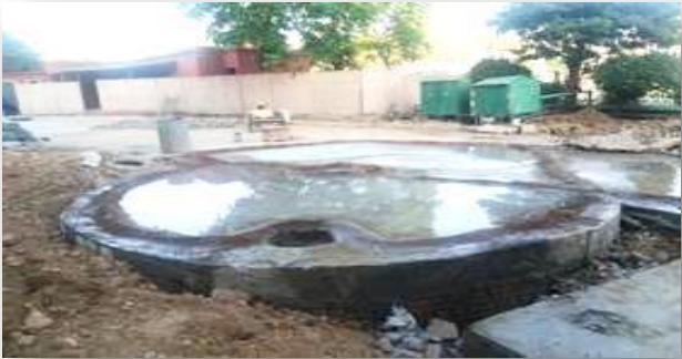
Rain water harvesting pits
